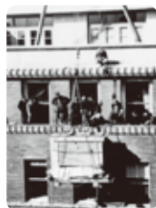
Installation of the UNIVAC120
