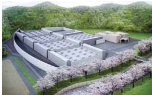
Obama Data Center
