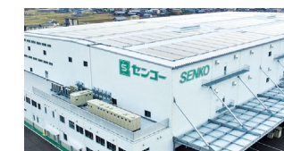
SENKO's Gifu-Hashima PD Center, introduced solar power generation equipment based on PPA and opened in May 2021
