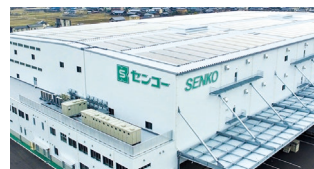
SENKO's Gifu-Hashima PD Center, introduced solar power generation equipment based on PPA and opened in May 2021
